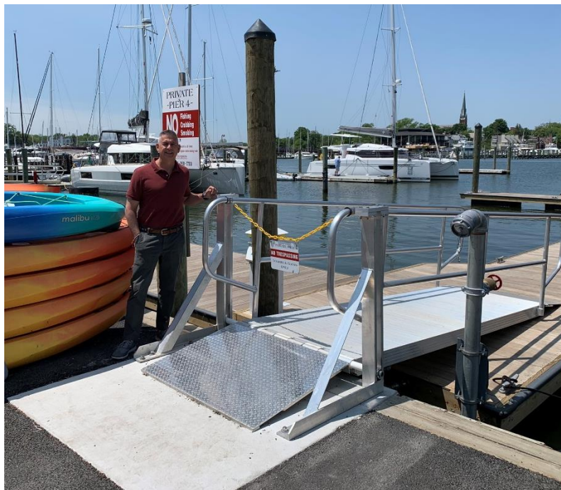
A view of the innovative levitating gangway and high pilings. Photo courtesy of Cardie Templeton, 2023.
