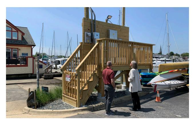
**4. Extra Long Feeds:** The electrical conduit and water lines from the bulkhead are one foot longer than they need to be to reach the pier at our goal height, which is also long enough to reach down to the dock if there's an equivalently extreme low tide.
